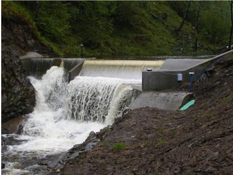
Intake weir showing trash screen (centre) and intake to pipeline (right)
