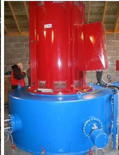
A 500kW turbine (blue) and generator (red)
