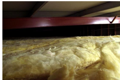
Figure 1 Typical loft insulation
