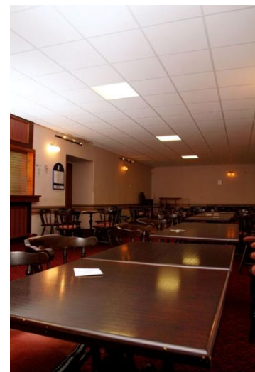
Figure 2- Example of newly installed lowered ceiling
